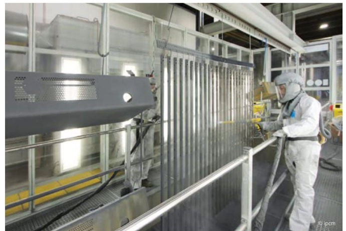
The powder application booth of the coating line for large parts.
